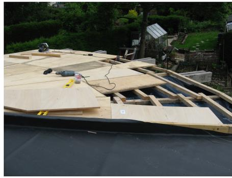
Plywood sheets being installed on the roof.
