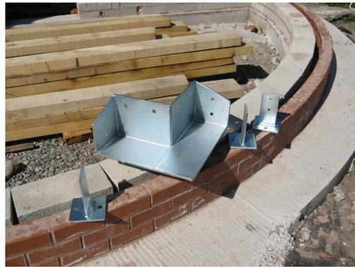
Straw bale extension base wall on concrete foundation with custom made galvanised brackets.
