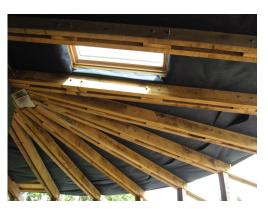
Internal view of completed rafters with roofing felt and skylight above.
