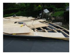
Plywood sheets being installed on the roof.
